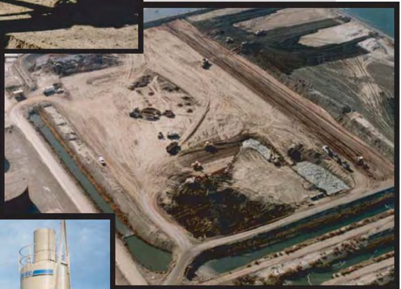
Stabilization of Refinery Sludge and RCRA Cell Construction
