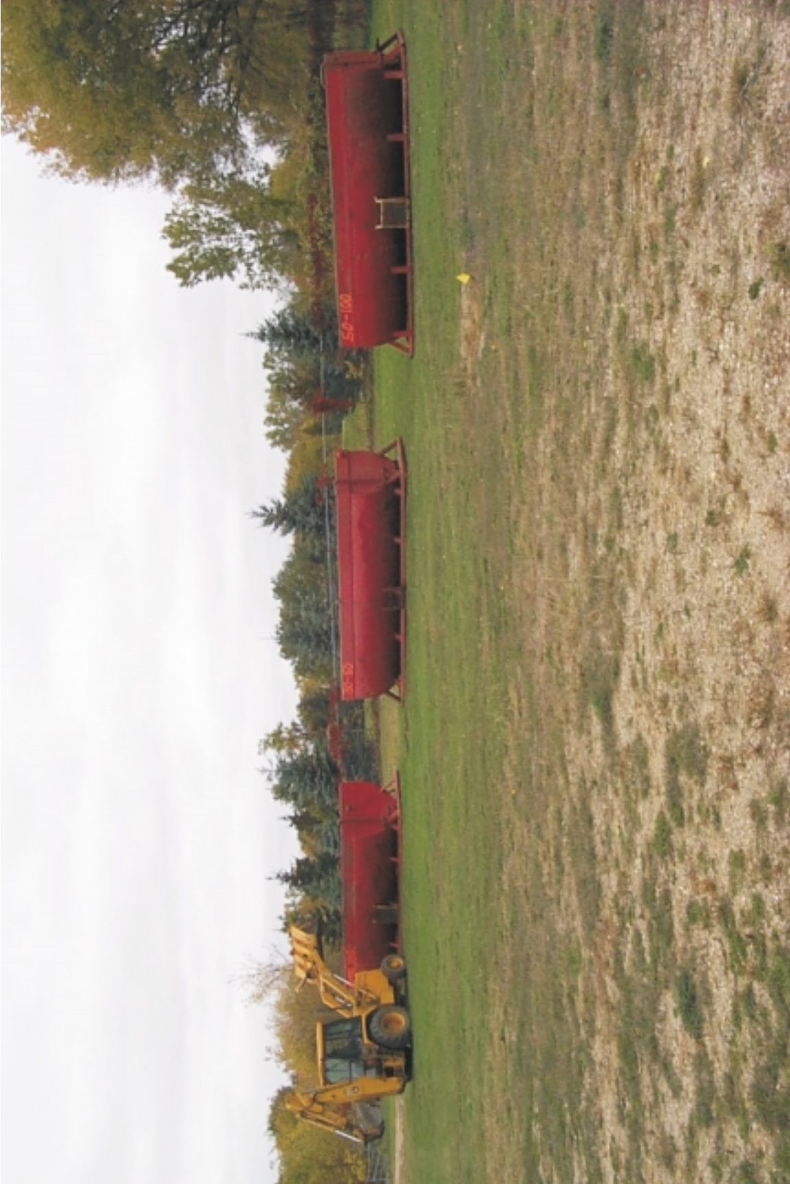
Figure 2.9 Segregation of Pan Soils into Storage Bins
